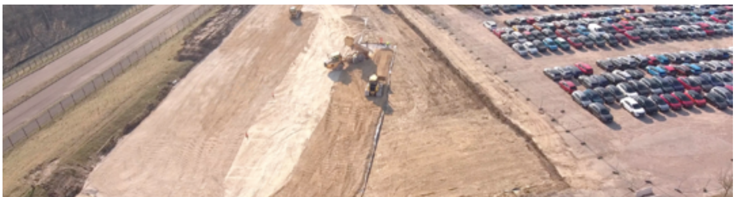
Drone footage of the ongoing earthworks in Rockingham
